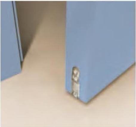
Automatic drop seal
