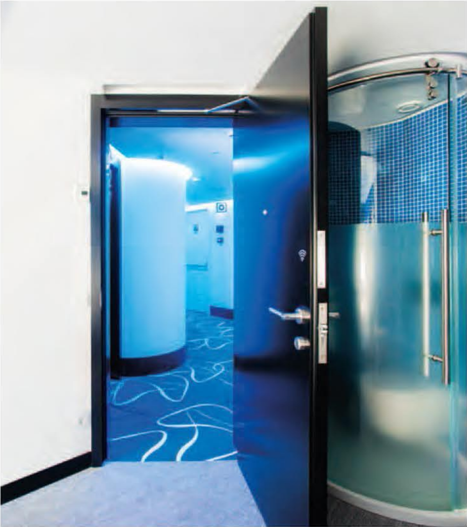
Rebated door with concealed door closer
